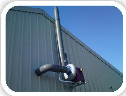
We control our fans with an inverter meaning the speed of the fan increases and decreases as required. This is a more energy efficient and therefore cheaper alternative to the antiquated way of using a damper within the duct.
