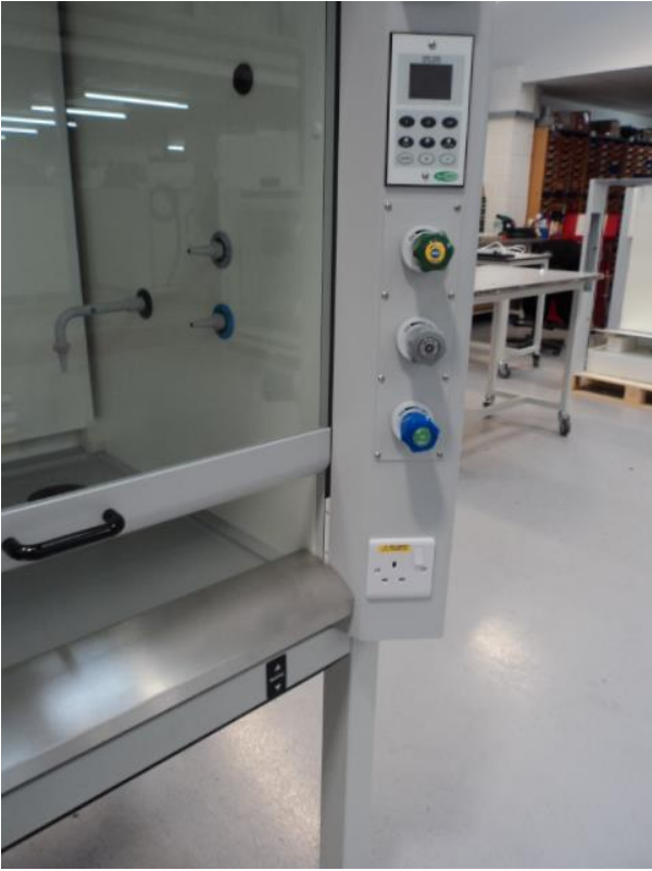
Airone XP: 54 VAV units, 4 with DDA compliant adjustable height stands
